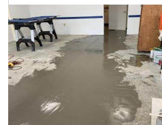
August 2020, Floor leveling
