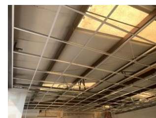
June 2020, Light fixtures started, and they look great
