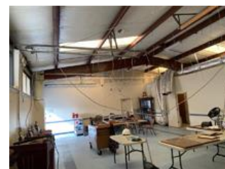
May 2020, Start of construction
