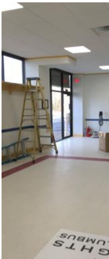
Doors and windows to be treated
